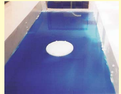
Tower basin after Pancrete XE applied
